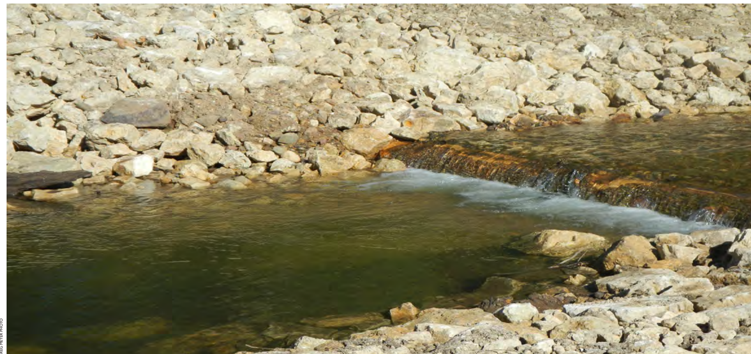
The first plunge pool installed at the headwaters of the Trimbelle
