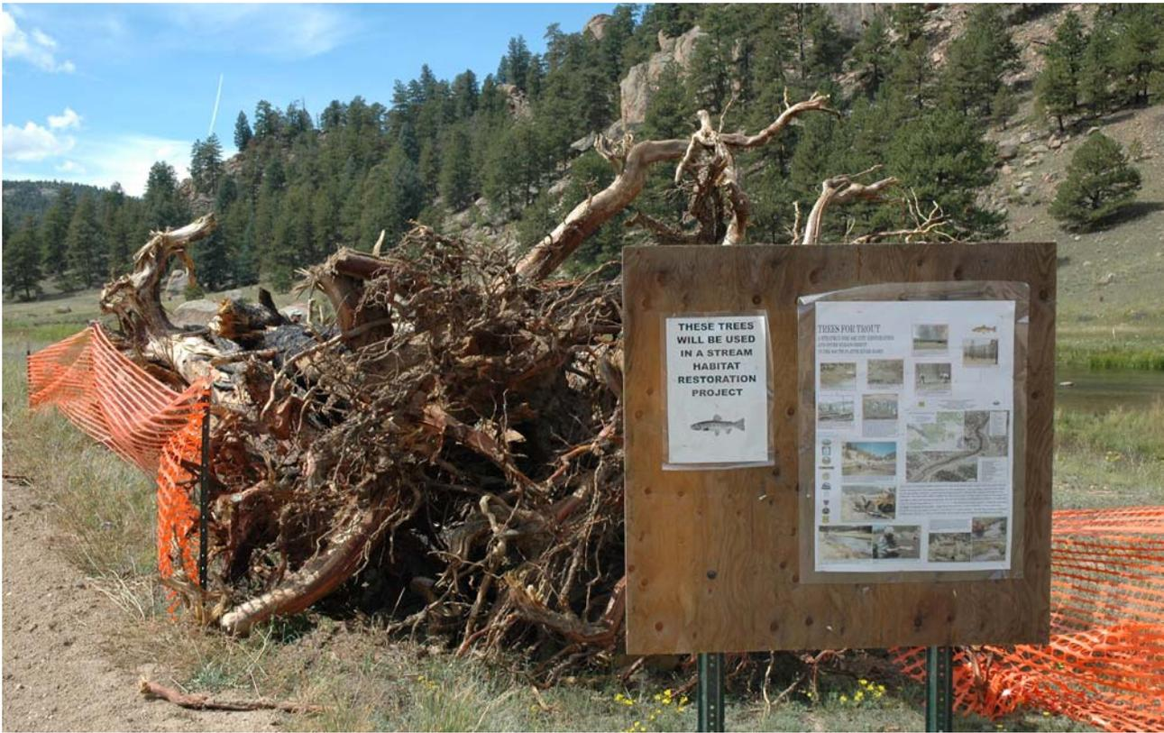
**Tree root balls like these were used to create trout cover in the Camp Alexander stream restoration project.**
